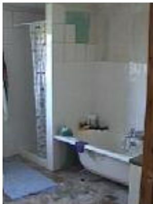
Marble on the floor and some tiles on the walls
