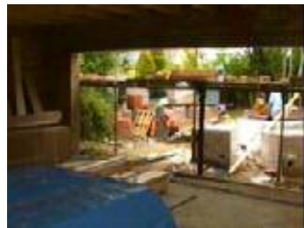
The view from the garage is still a building site!
