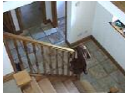
Slate on the hall floor is still being grouted
