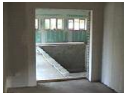
The pool is screeded
