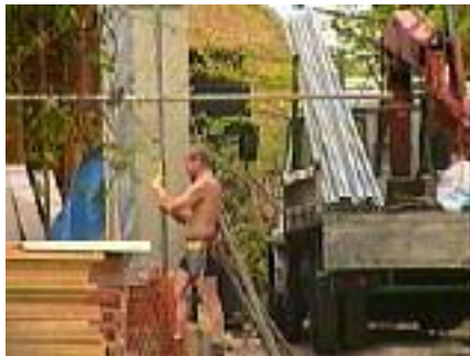
We arrived to see the scaffolding going up.
