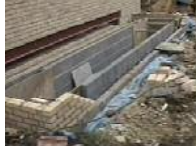
The pool cover pit progresses
