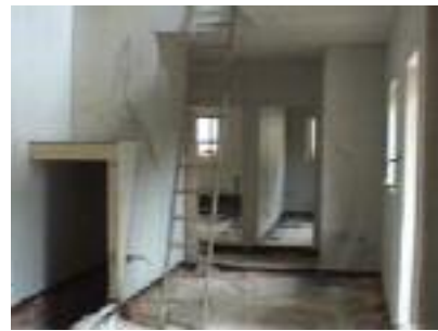
There were rooms upstairs
