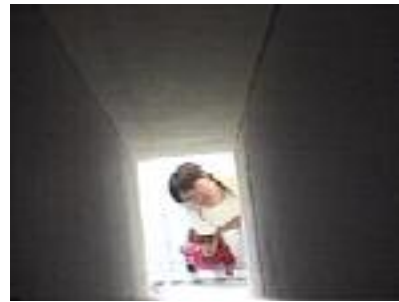
The laundry chute
