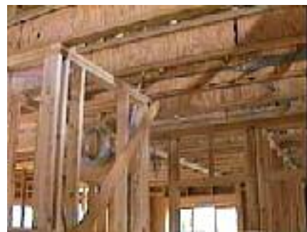
We sprout security and mains cabling.
