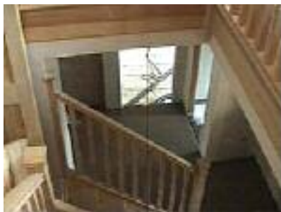
The hall is screeded
