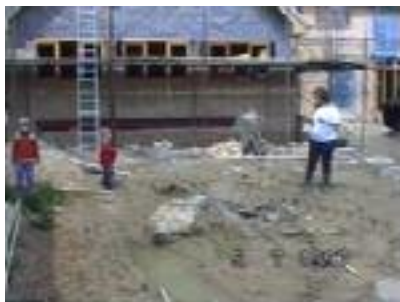
In just a week the roof had been set and tiled, and the windows were in so the brick layers could work up to them
