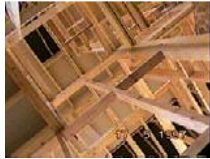
The stairs for the staff quarters arrive and decking is laid in the attic to make sure no-one lays cables or pipes into the loft because they don't expect there to be a floor. The view from the basement straight up through the loft hatch is a longggg way!
