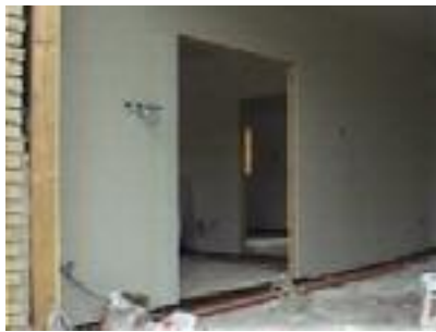
The dry lining went in in just a few days
