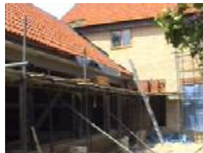
In just a week the roof had been set and tiled, and the windows were in so the brick layers could work up to them
