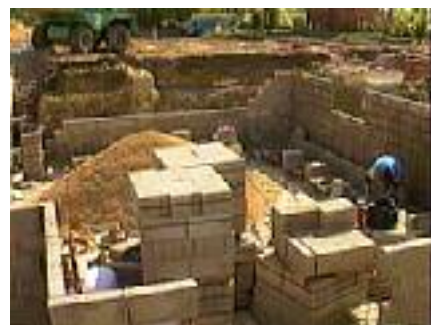
The next time we saw the plot, the brick layers were busy bringing the foundations up to damp proof course level. The cellar walls were being built. Two layers of breezeblocks with reinforcing steel in between. The gap is then filled with concrete.
