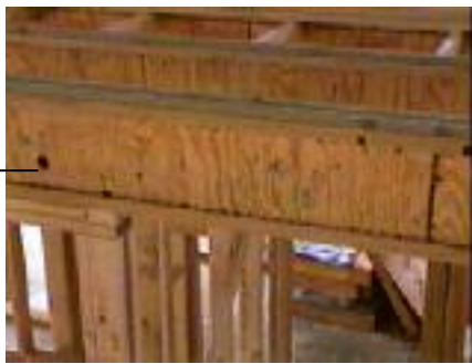
The floor joists have pre-stamped holes which simply have to be knocked through so wiring or pipes can pass through.
