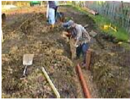
The first thing to be done was to build the drains.
