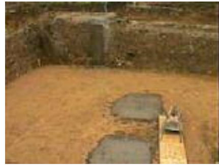
Then the cellar was dug
