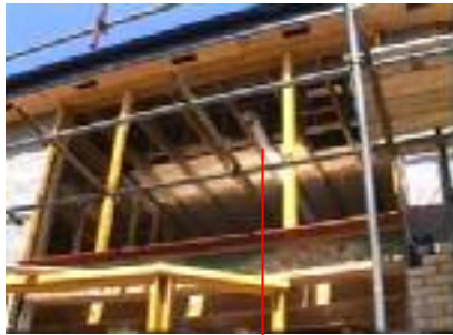
Heat exchanging ventilation
