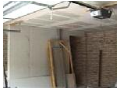
The garage door and opener is fitted
