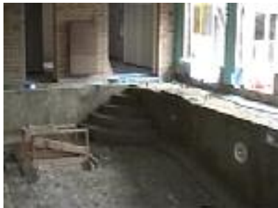
The pool gets its lining undercoat skim
