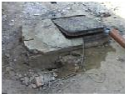
More pumping with the pipes wedged
