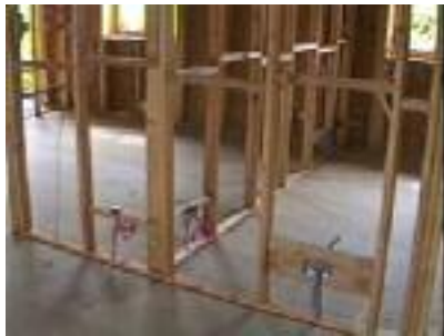
At last a floor! The cabling began to find a home too.
