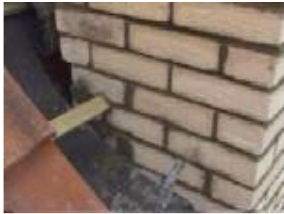
The chimney was sorted out
