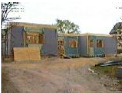
It's really beginning to look like a house.
