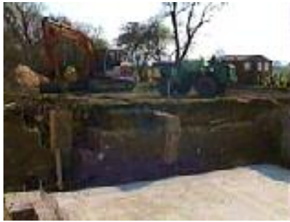
When we came the following week, the cellar had a concrete base, the kitchen and dining room had foundations and the spoil heap had been levelled out.
