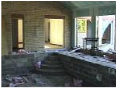
No scaffold in the pool.
