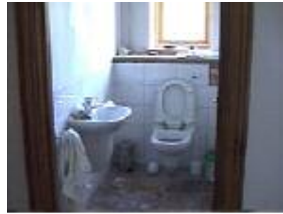
Wood stain on the door frames, most of the bathrooms work now.
