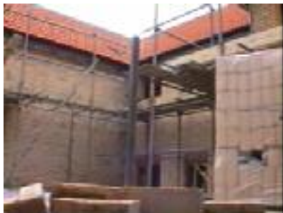
The bricks were getting to the top
