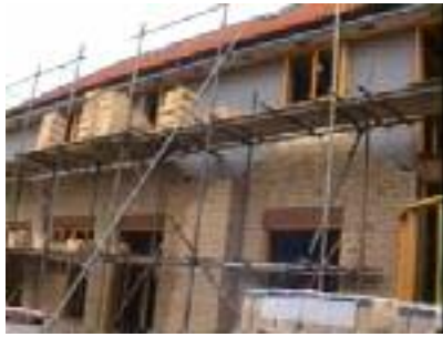
The bricks were going slowly
