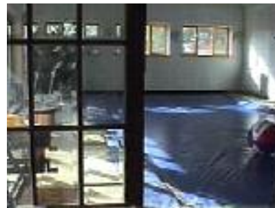
We're still laying the slate in the pool room. The pool cover is on.
