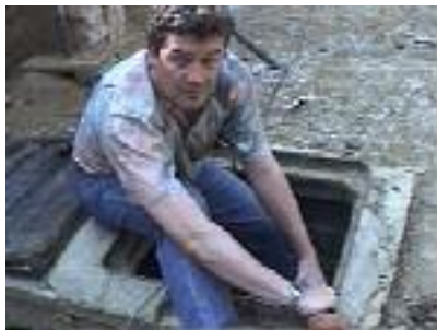
Someone has to hold the pipes in place
