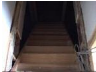
The stairs went down as well.
