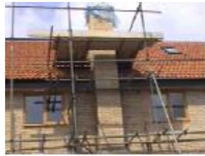
The scaffold is coming to the top
