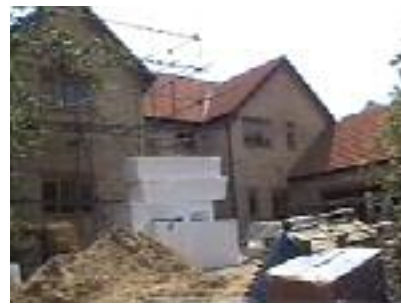
Some of the scaffold comes down
