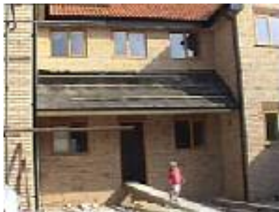
The front door has a canopy but no step
