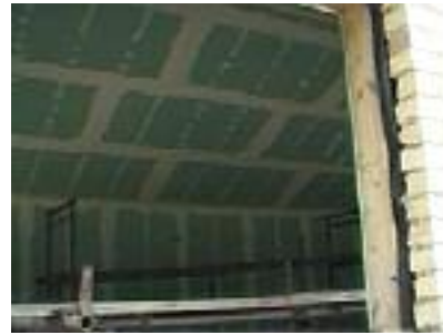
The pool gets its dry lining
