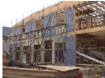
The roofers and brickies will use the scaffold.
