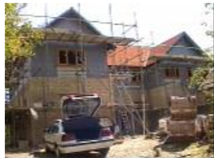
A week later the progress is steady.
