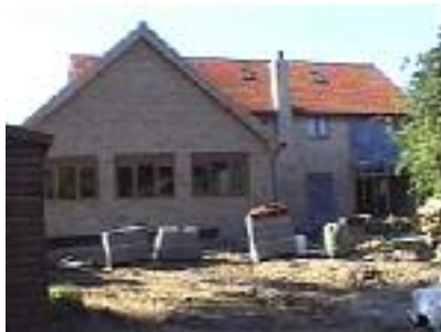
Still a building site
