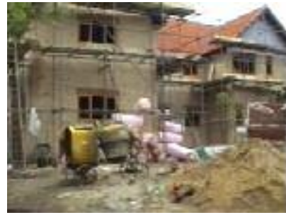
but progress was being made.
