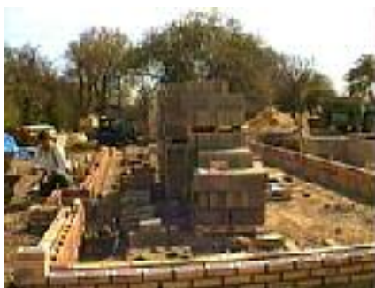
The next time we saw the plot, the brick layers were busy bringing the foundations up to damp proof course level. The cellar walls were being built. Two layers of breezeblocks with reinforcing steel in between. The gap is then filled with concrete.
